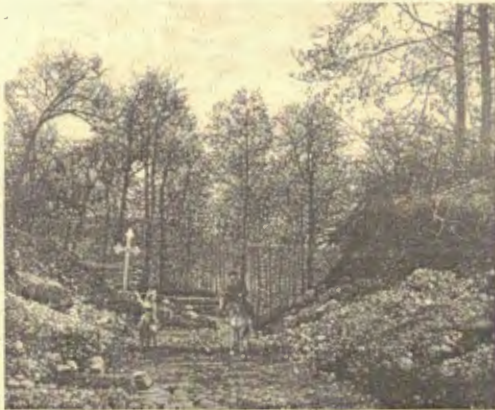
Stations Way: An Earth-Cut On The Ascent 25
